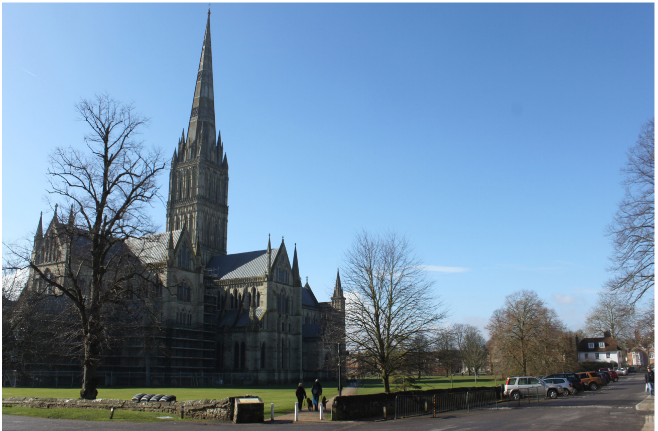
Image 3: Existing pathways lead visitors to the North Porch
