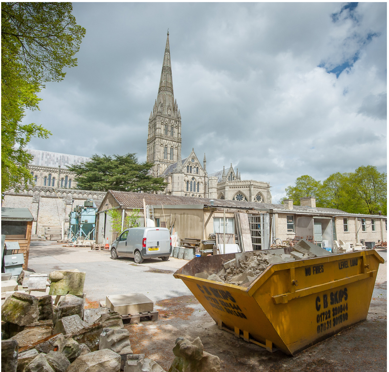
Image 6: The existing Works Department
